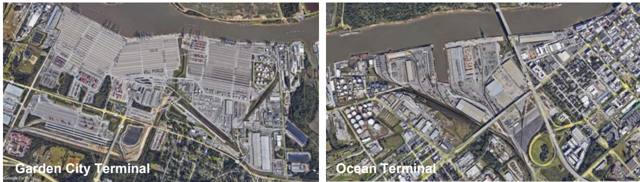
FIGURE 4.1 DEEPWATER TERMINALS AT THE PORT OF SAVANNAH
